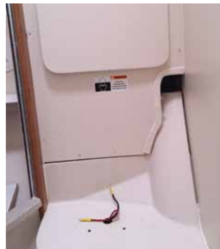
Toilet removed with sufficient length wires to be reconnected.
