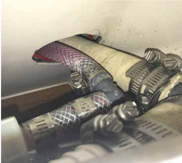
Hole behind toilet was drilled to accommodate both discharge hose and water line.
