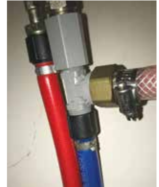
T connector to freshwater line.
