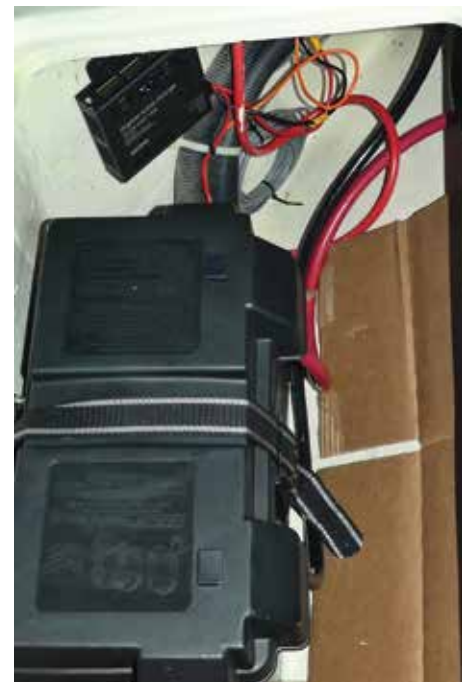
The SG200 was placed above the switch panel and utilized an existing cut out in the top back of the panel.
