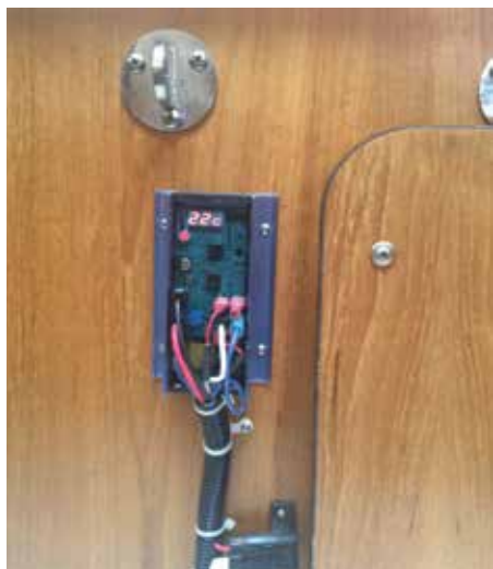
Balmar ARS-5 installed below the stairs.
