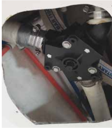
Hole cut in cabinet wall revealing location of the new valve.
