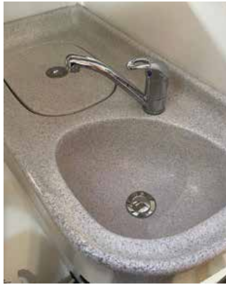
New sink drain install
