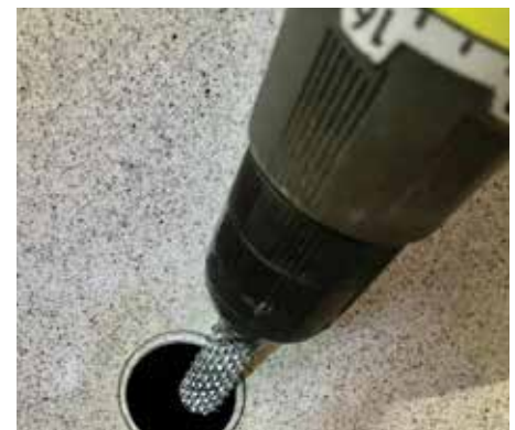
Enlarging sink drain hole
