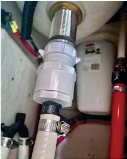
New sink drain connections
