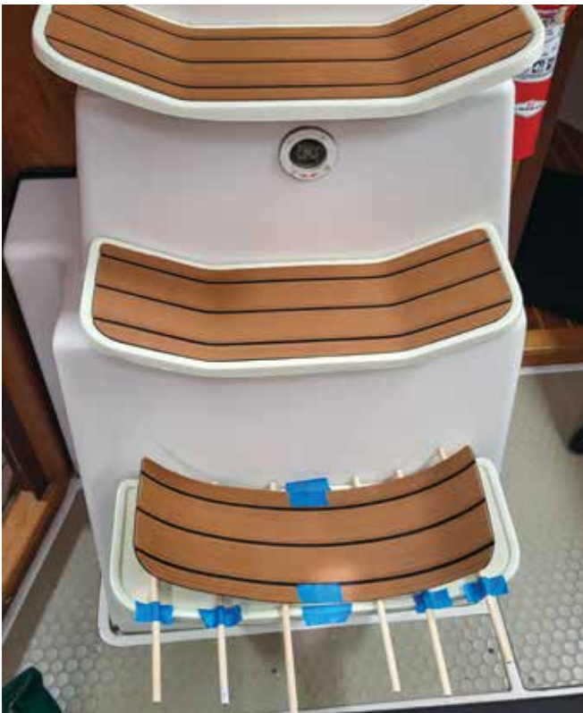
New insert cut and ready to align
