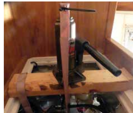
The bottle jack on the 2x4 that was held in place so it would not move
