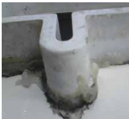
Old Sealant Under Rain Drain Lip
