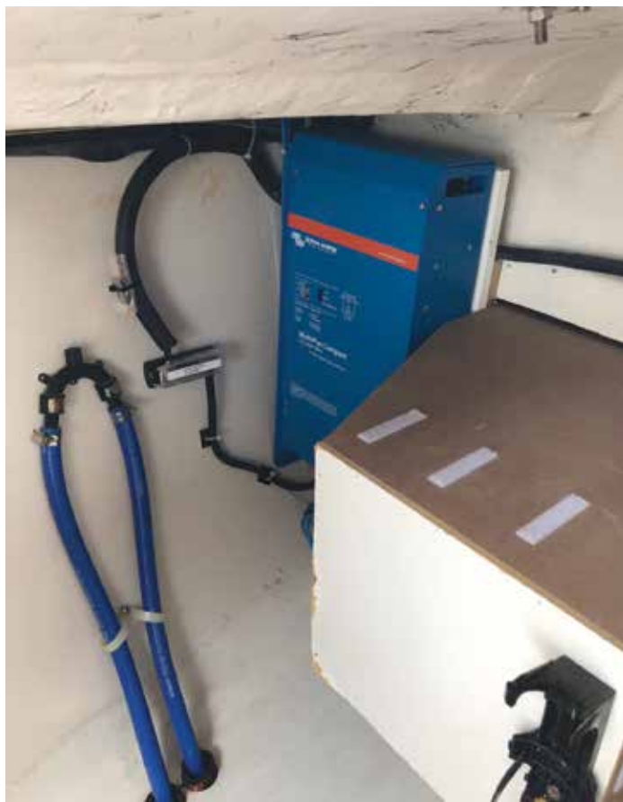
Installed Multiplus
