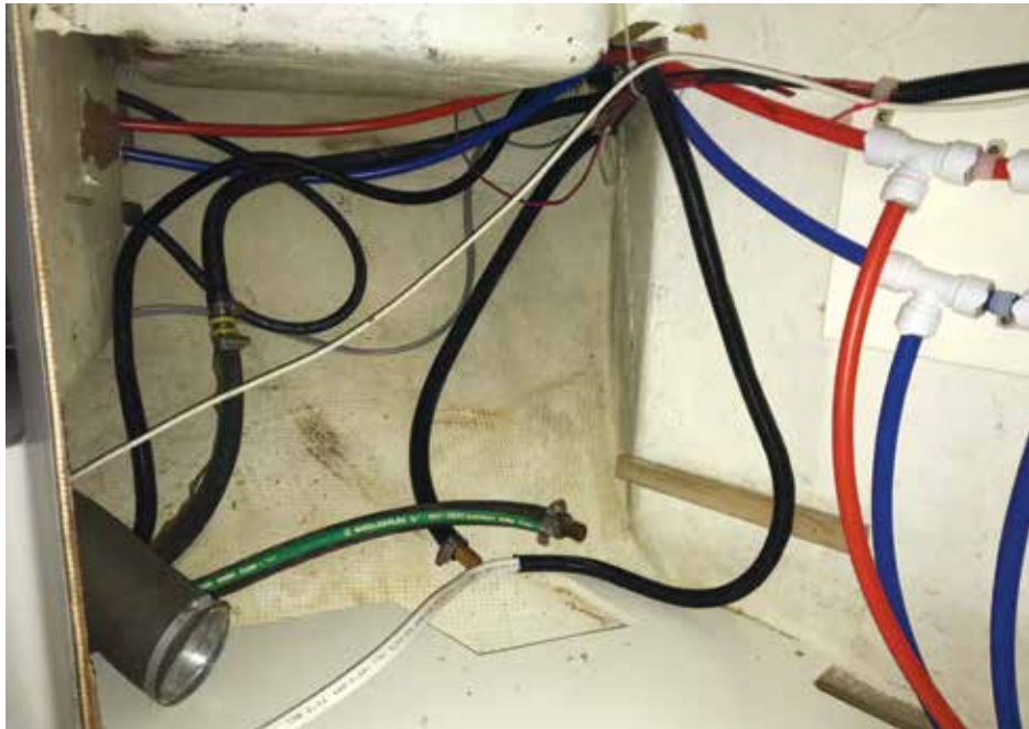
Water heater and supply pump removed and the beginning of the new PEX manifold. Note the engine heat hose running to the upper right - this would go away as part of project creep.
