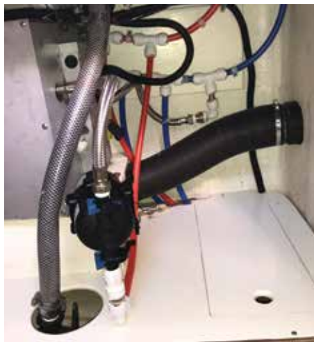
New water heater installed and the PEX supply manifold complete. The small, black tank in the center foreground is an accumulator tank.
