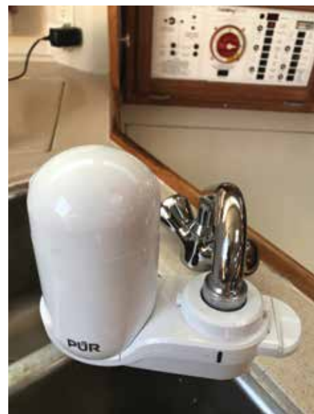
PUR water filter on galley sink faucet. Note small, flat switch at right of filter. In this position, water bypasses filter. Move switch down for water to pass through filter.
