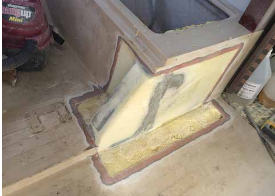
Pourable Foam Fills Voids, and Makes for Nice Surfaces for Finishing
