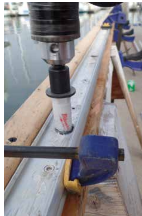
Drilling new extrusion through hole in old
