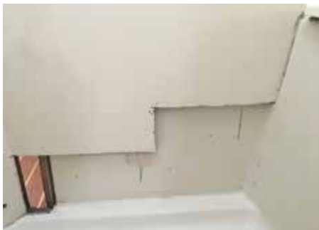
Excised section of bulkhead; cut back to sound material.
