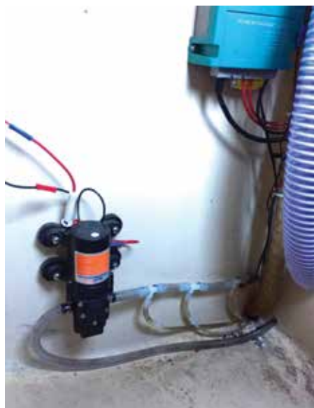
DIY Arid/Dry Suction Manifold and Diaphragm Pump
