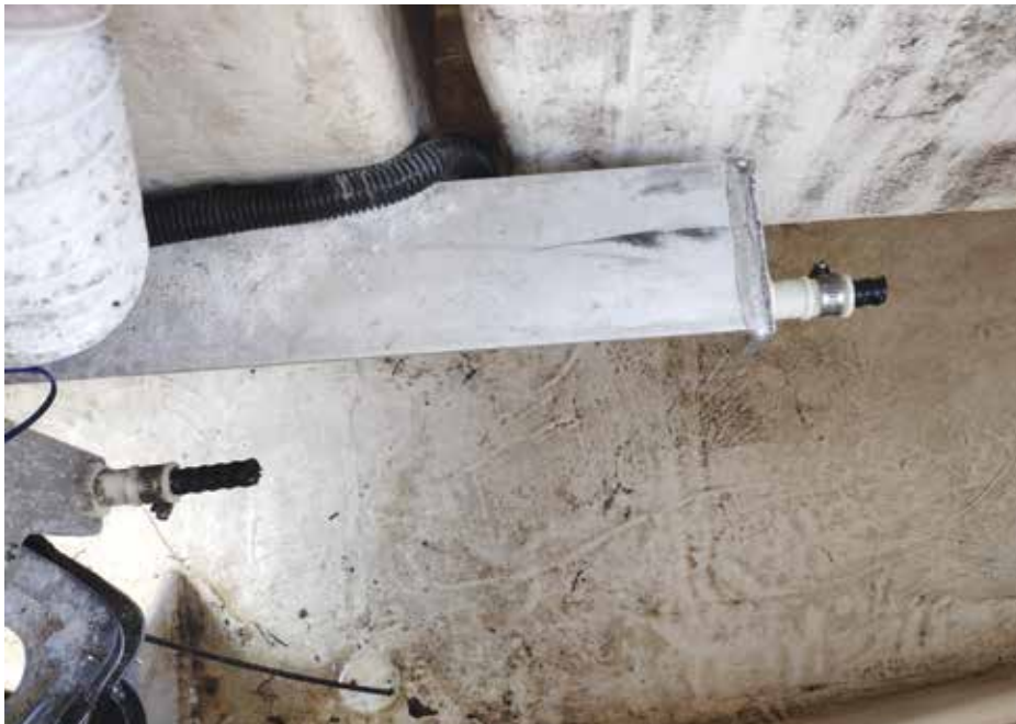
The old conduit and chain removed with a cutting wheel
