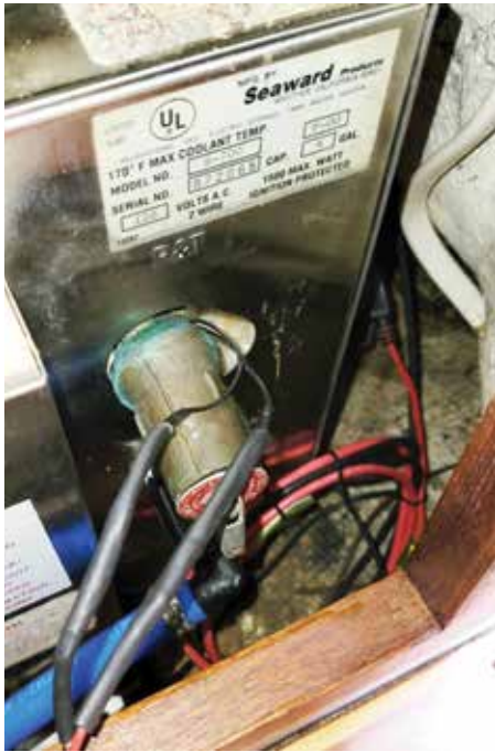
The hot water probe inserted between the tank and the insulation
