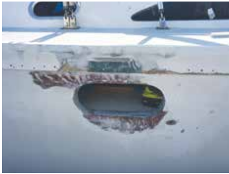
Fiberglass repairs begin
