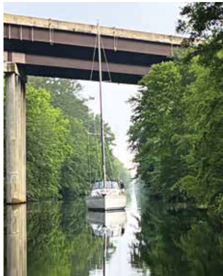
We made it! We successfully passed under our first 65ft bridge.
