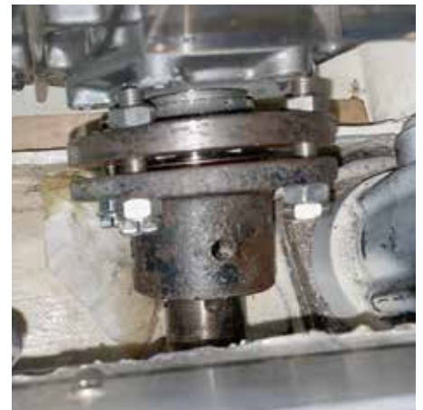
Original prop shaft collar and engine attachment showing problematic bulkhead
