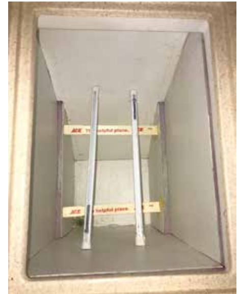
Adding FRP Facing
