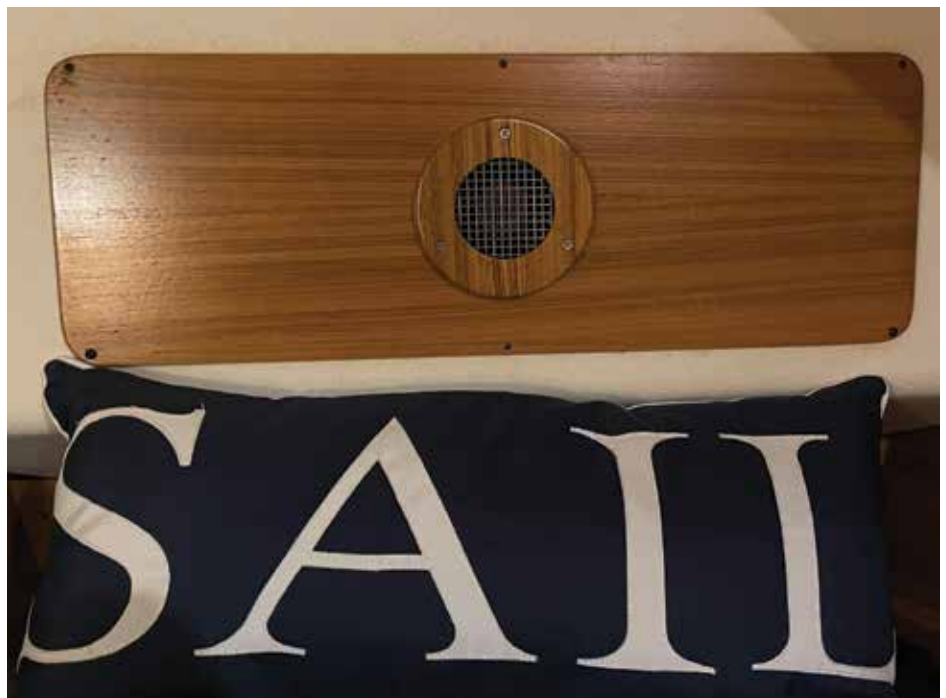
Forward Cabin Fan Installed
