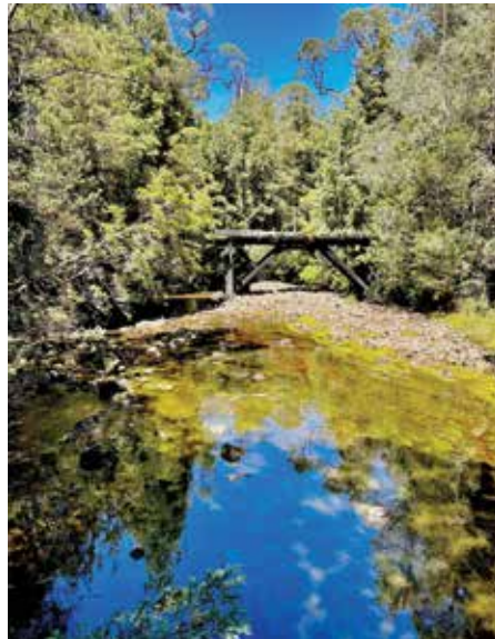
Bird River Bridge
