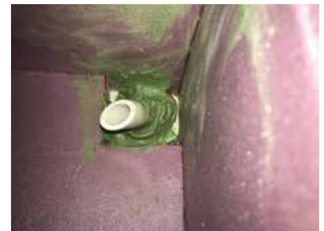
Drain Modification prior to 2nd layer of foam
