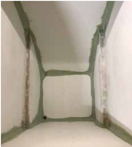
Finishing the corners
