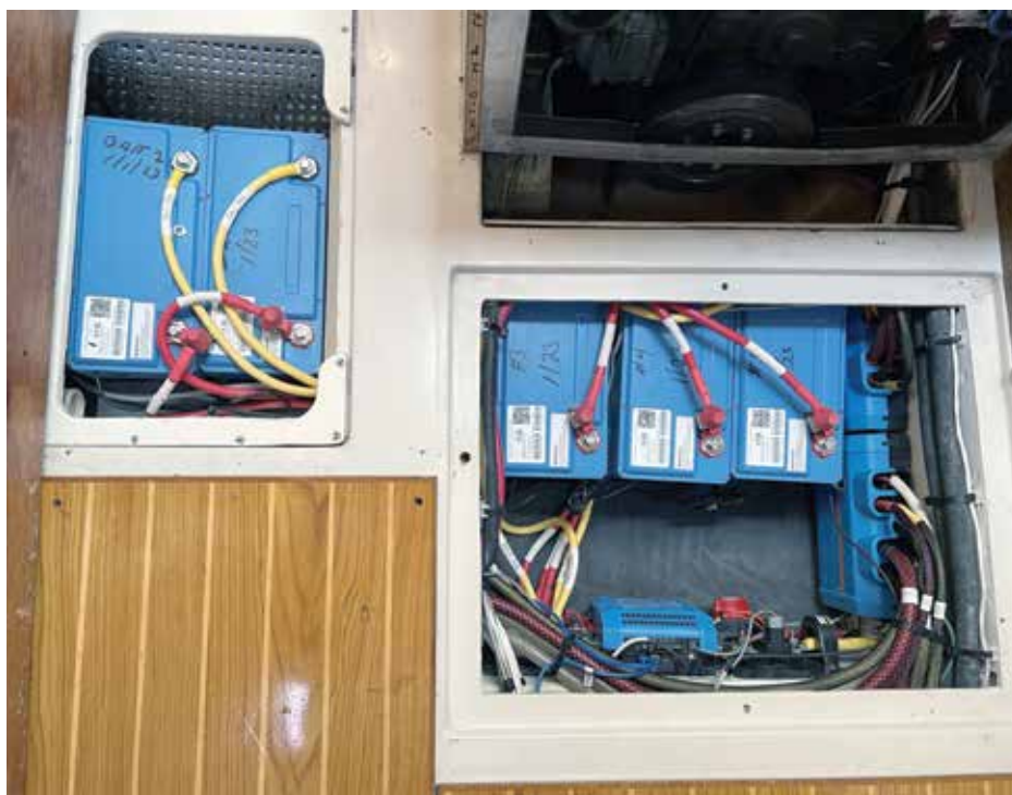
Installation of Dulcinea ’s LFP batteries and control modules
