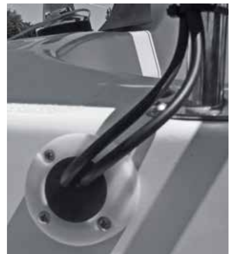
Solar wires led through the cable gland into the port quarter locker.
