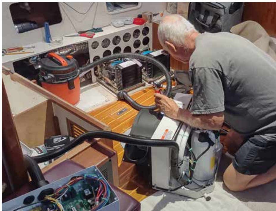
Replacing the salon/forward air conditioner. Photo by Julie Lynn Olson.
